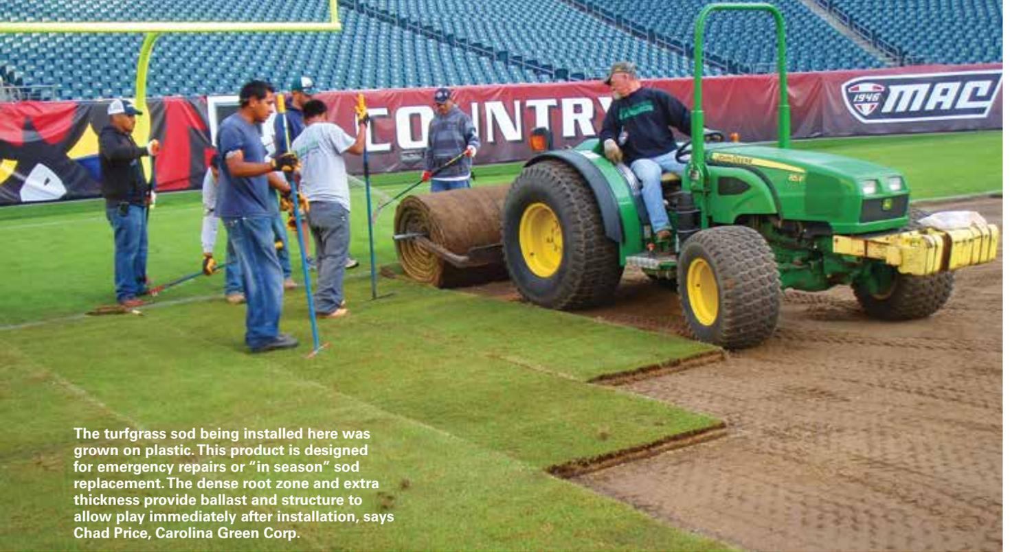
The turfgrass sod being installed here was grown on plastic. This product is designed for emergency repairs or "in season" sod replacement. The dense root zone and extra thickness provide ballast and structure to allow play immediately after installation, says Chad Price, Carolina Green Corp.
