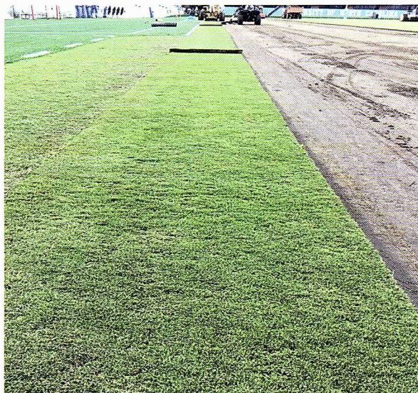
Installing the new sod.
