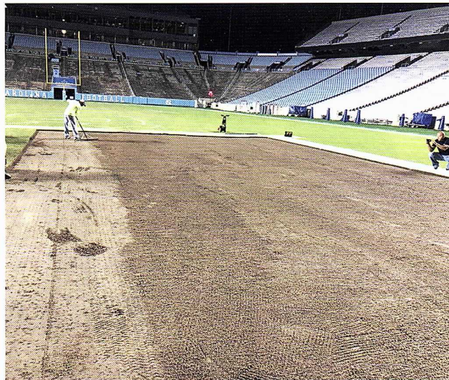
Field area preparation for a partial resodding.
