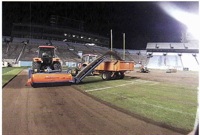
Removing the old sod.
